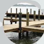
Marine construction and bridges
